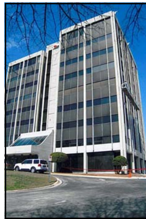
Front of building—OLD
