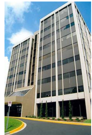
Front of building—NEW
